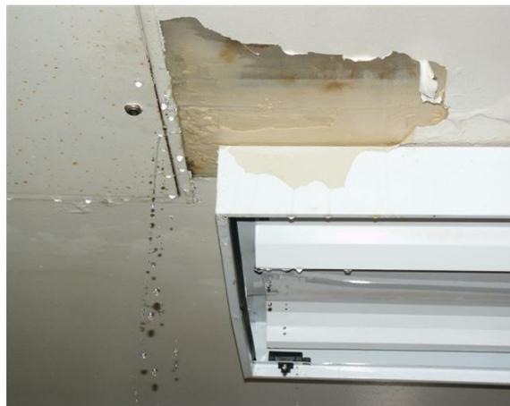
**Figure 4 – Water leak in light fixture. Photo: CCWF Plant Operations**
